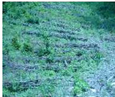
Figure 2. Wattle fences: a. application of the slope; b. a slope arranging with wattle fences
