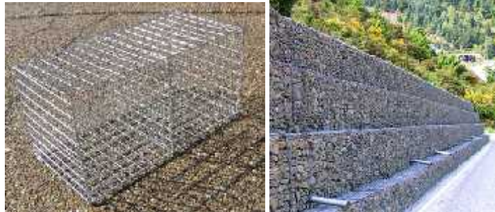
Figure 3. Gabions: a. gabion structure; b. a slope arranging with gabion Source: a. http://www.gabionbaskets.net ; b. http://www.gabionindia.com
