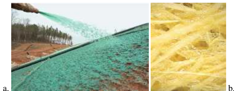
Figure 7. Soil Guard: a. application of the slope; b. fiber matrix Source: a. [54]/ b. www.emeraldseedandsupply.com
