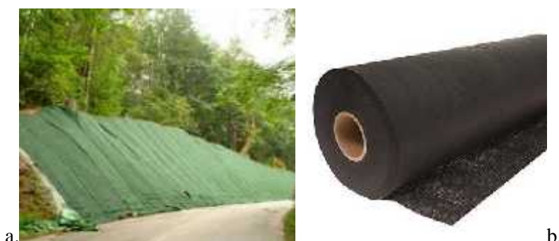
Figure 8. Geotextiles: a. Application of the slope; b. geotextile roll Source: a. http://your.kingcounty.gov/kcdot/roads/cip/ ; b. www.google.ro/search?q=geotextiles+roll&biw
