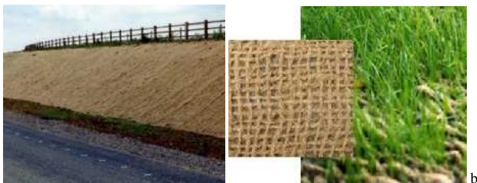
Figure 6. Nets biodegradable jute; a. application of the slope jute; b. detail jute Source: a. www.hy-tex.co.uk / b. http://www.ecomerchant.co.uk
