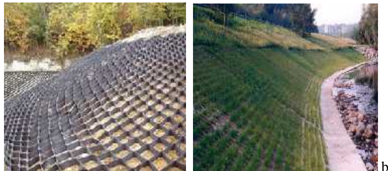
Figure 4. Cellular paving with grass: a. application of the slope; b. a slope arranging Source: a. http://www.terram.com ; b. http://www.sustainablepavingsystems.com
