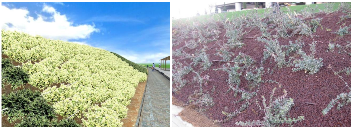
Figure 7. Slope stabilization with a) 3D modeling of slope; b) slope in situ Source: Original Photo
