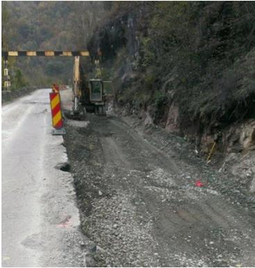
Figure 1. Excavation of roadside box
