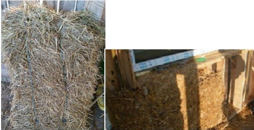
**Figure 1.** Straw bales used for thermal insulation in the Transylvanian Plain
