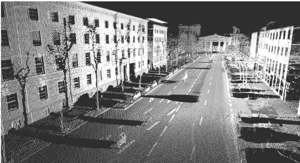
Fig. 4 - Example of "point cloud" obtained from a kinematic scan in Munich [Kinematic 3D Laser Scanning for Road or Railway Construction Surveys – G.GRÄFE]
