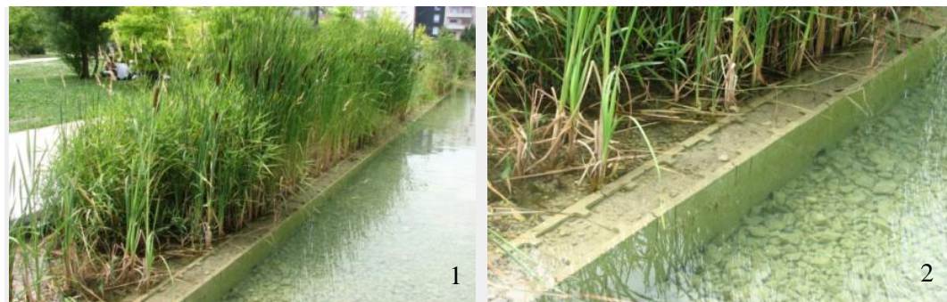
Fig. 2. Constructed wetland: 1. wastewater filtration tank; 2. construction detail (original)
