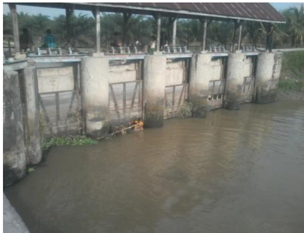
Fig. 2. Installation of Irrigation in Rawang Panca Arga Subdistrict
