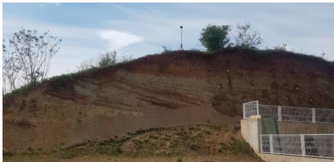
Fig. 1 Tilting the slopes on the slope
