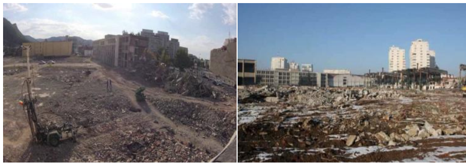
Fig. 9. The current situation of the site
