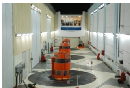
Figure 2. Mărișelu Hydroelectric Power Plant
