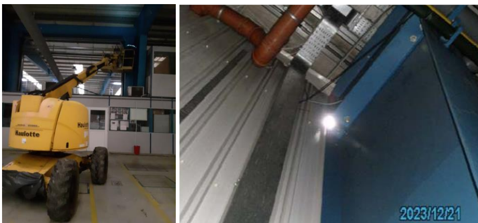
Fig. 3 Fixing reflective targets
