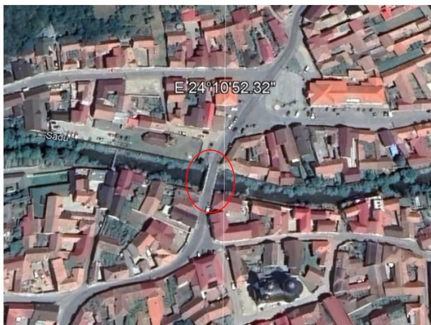
Fig. 1 Location of the studied bridge
