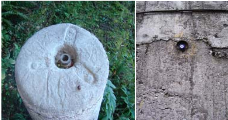
Fig. 4. Pilaster with clamping device
