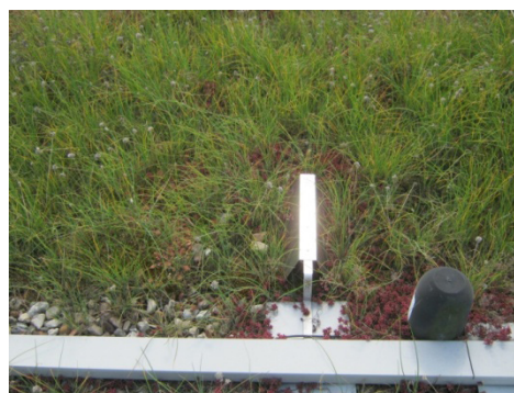
Fig. 6 Log 32 placed on the green roof Source: original
