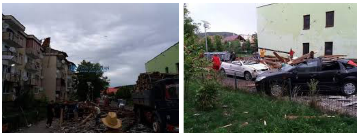
Figure 3. Damage produced in Aghireșu area after strong storm and wind
