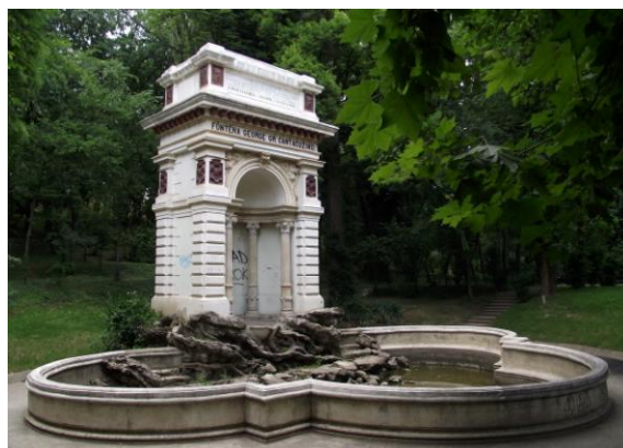
Fig. 2. Cantacuzino fountain in Carol I park, June 2011
