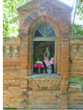
Fig. 10. Minute church as a part of stone wall; Source: Gabrijela Jurić, 2009
