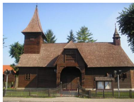
Fig. 2. St. Barbara chapel in Velika Mlaka Source:hr.wikipedia.org/
