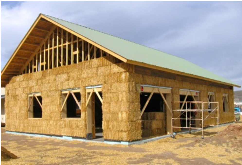
Figure 2. Construction with load bearing straw bale structure [21]
