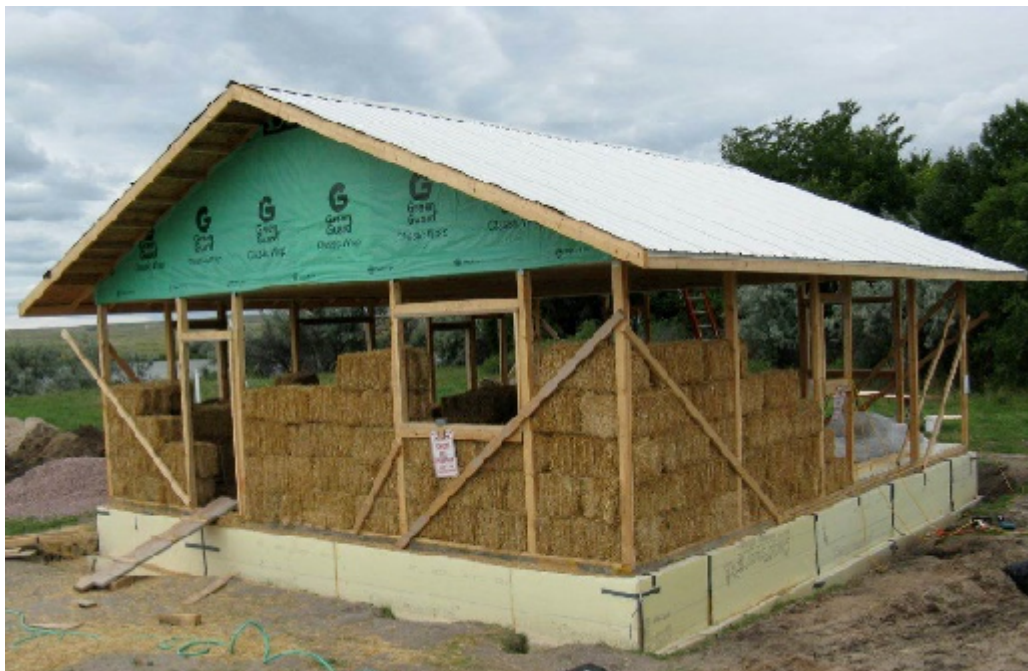
Figure 3. Straw bale construction with timber frame structure [20]
