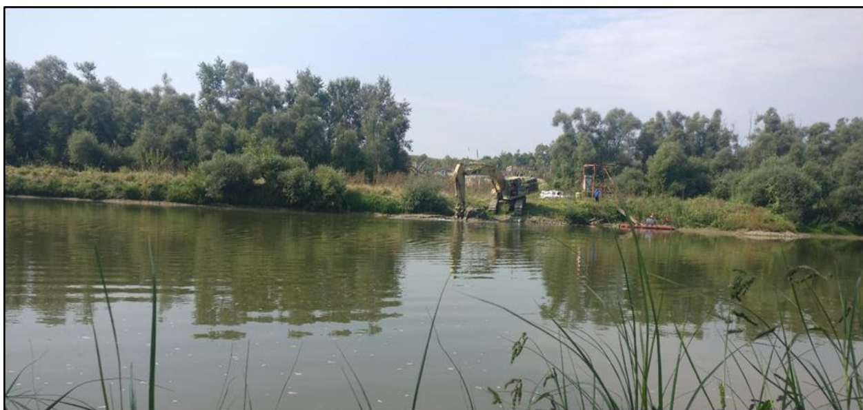
Figure 3. Silt deposits from quarry water leakage in Someș River being excavated in sampling point 3.
